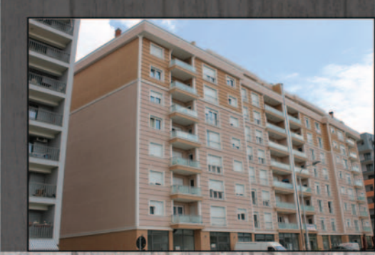
Kompleksi Trio Construction Lagjja Kalabri
